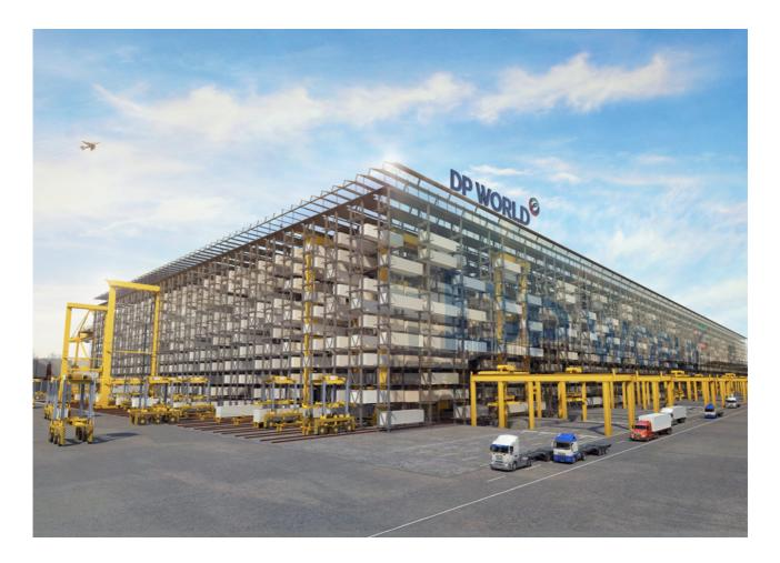
BOXBAY by DP World offers new solutions for container storing and handling through its High Bay Storage (HBS) system. Using a system such as this can free up much of the space required. As an example, Dublin Port is made up of 260 Hectares of which approximately 12% is used for container and container management. This equates to 31 Hectares and by using an automated system will leave 25 Hectares available for uses such as the Eirgrid Sub Station.
